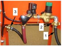
Fig. 42: Disconnecting the water supply
