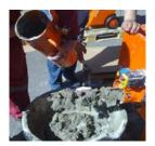
**1.** Clean the mixing tube and mixing shaft.
